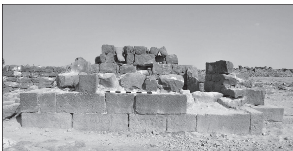
5. West façade of North Tower with only remnants of the lower two courses remaining. 17 June 2015. (photo: Bert de Vries).
