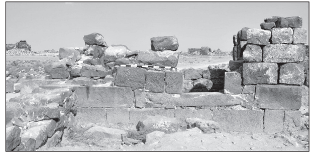
14. West façade of the Commodus Gate South Tower before preservation. The wall in the bottom left corner of the photo is the West Church courtyard wall constructed in the 6 th century. The doorway to the right of the scale stick was also inserted in the Byzantine remodeling to adapt this tower room as a churchyard outbuilding. 17 June 2015 (photo: Bert de Vries).
