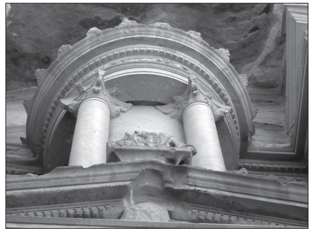
79. al-Khaznah. Tholos and lower pediment cornices.
